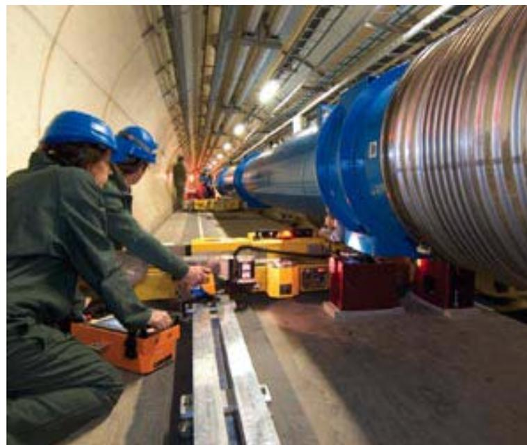
First dipoles being installed in the LHC tunnel on March 7 2005.
